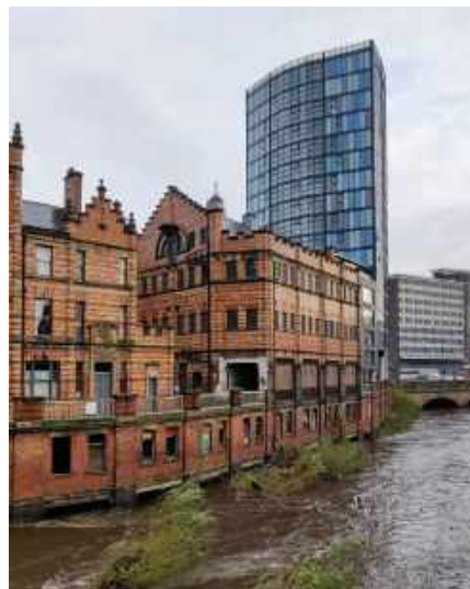
Royal Exchange Buildings, The Wicker
